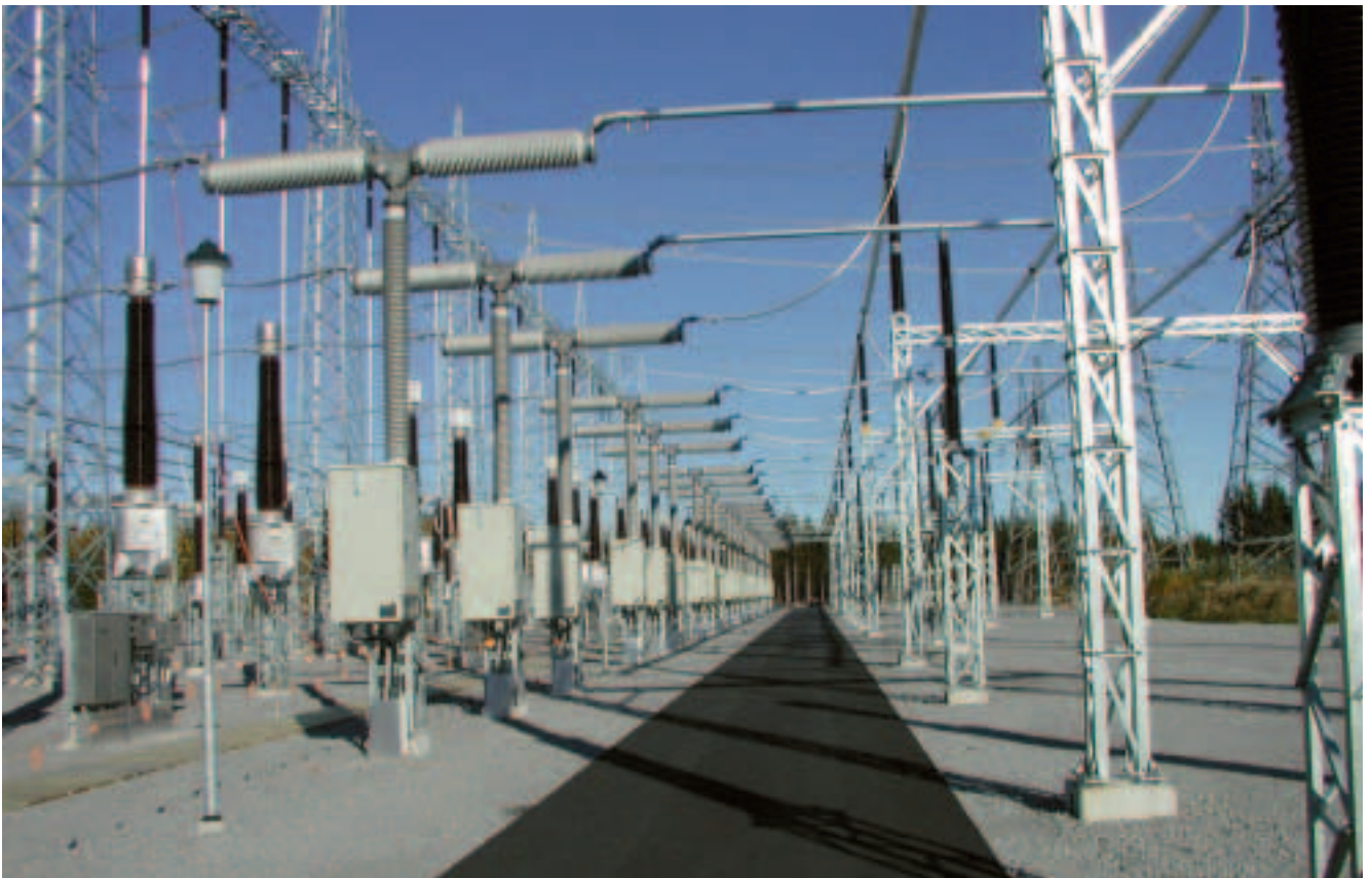
The Combined circuit-breaker, that ABB has developed in collaboration with others, including Svenska Kraftnät.
