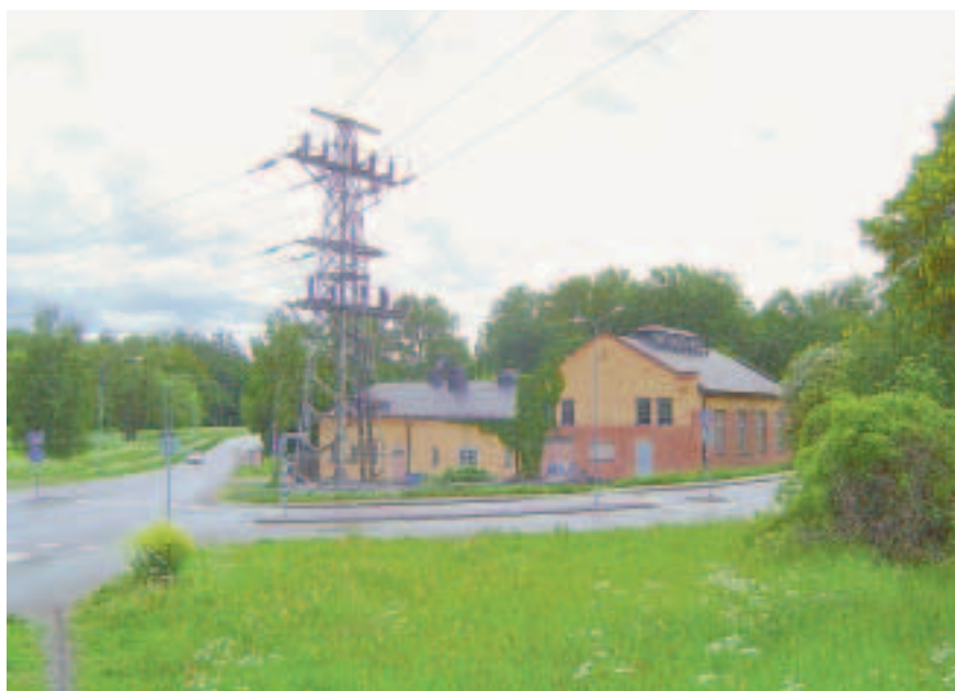
70 kV powerlines at Lidingö's first power station will be replaced by a buried 220 kV cable.
