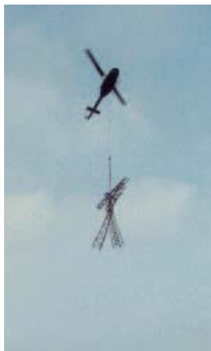
During the dismantling of a 220 kV line, the pylons were flown by helicopter to a specially-prepared site ...
