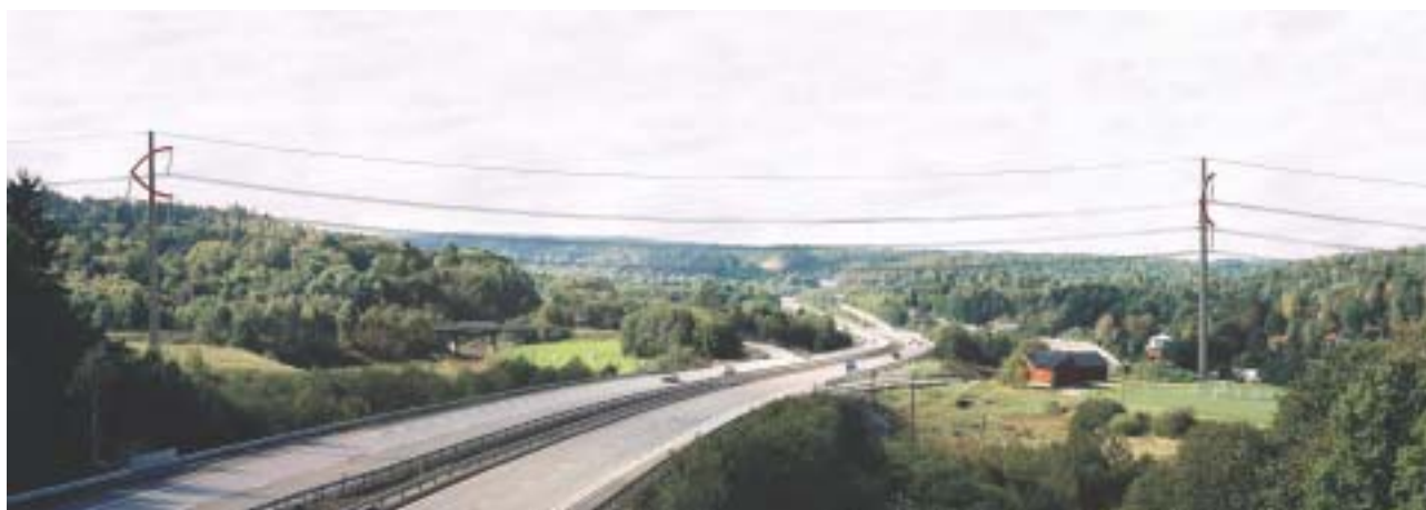
Svenska Kraftnät is planning to build a new 400 kV line between the stations at Stenkullen and Lindome, in the Gothenburg area. When crossing trunk road 40, one alternative would be to erect the line using specially designed compact pylons, which are well-suited to the environment in question (composite picture of design pylons in situ). See also the above picture.
